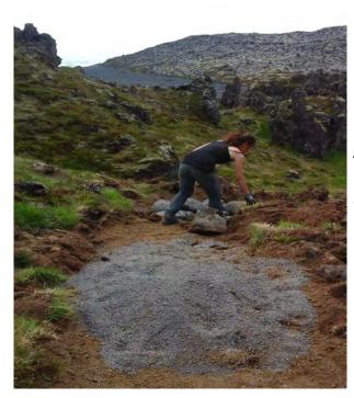
The paving stones, which are plentiful in this area, are laid on a bed of gravel, which is spread in the bottom of the path tray.
