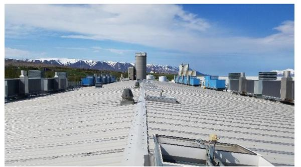
**Picture 2-6:** Exhaust units on the roof
