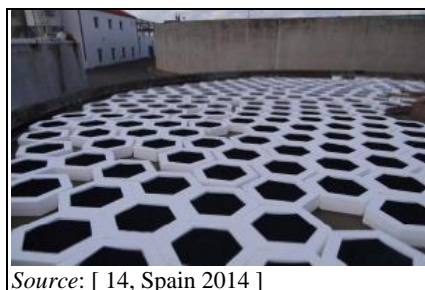
Figure 4.78: Geometrical plastic tiles in a slurry tank
