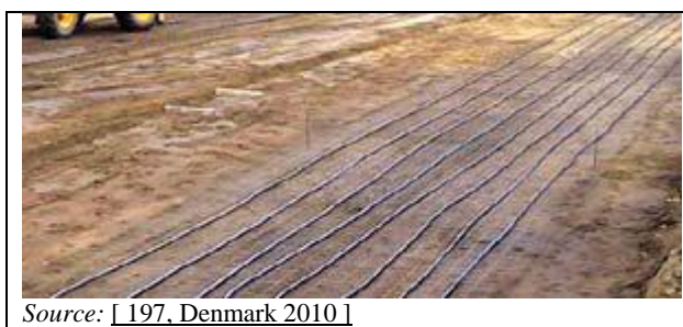
Figure 4.30: Example of PE pipes ready to be cast in concrete
