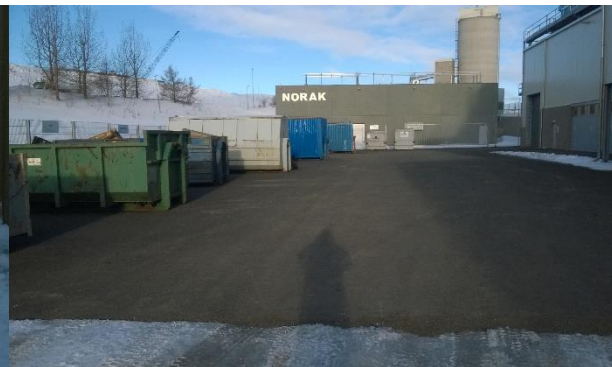
Picture 2-4: Measurements at the container area
