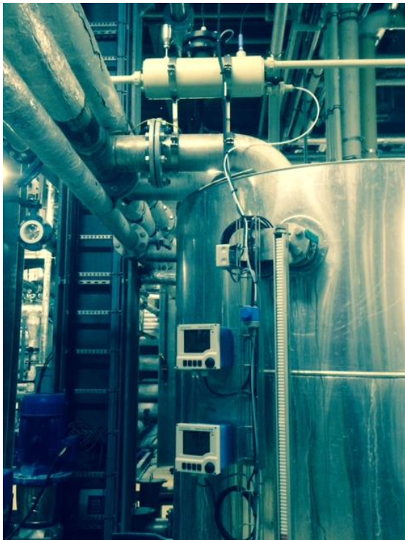
Picture 2-2: Temperature- and pH-meters for the measurement of Preox
